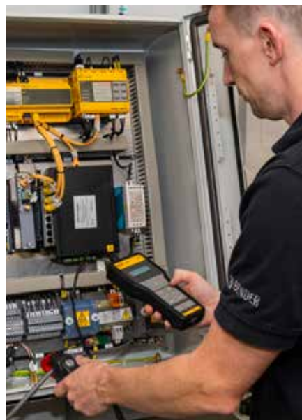
Final testing of rail equipment Protecting the health of electrical infrastructure is at the core of Bender UK's activity in the UK and Ireland. The company works with consultants, OEMs and end-users to deliver solutions
